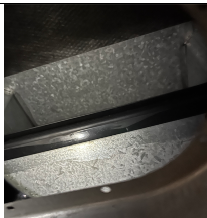
16. Partially open damper, no modulation
