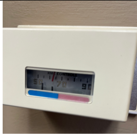
2. Typical localized T-stat for control, No BAS control
