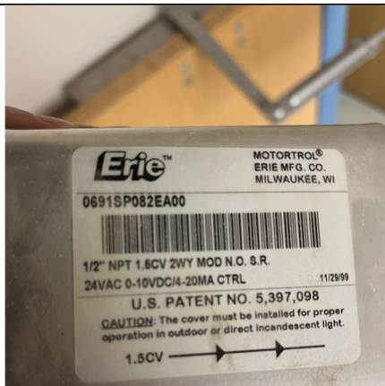
17. Typ control valve nameplate
