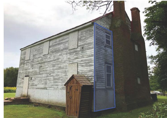
WEST GABLE END WALL:
