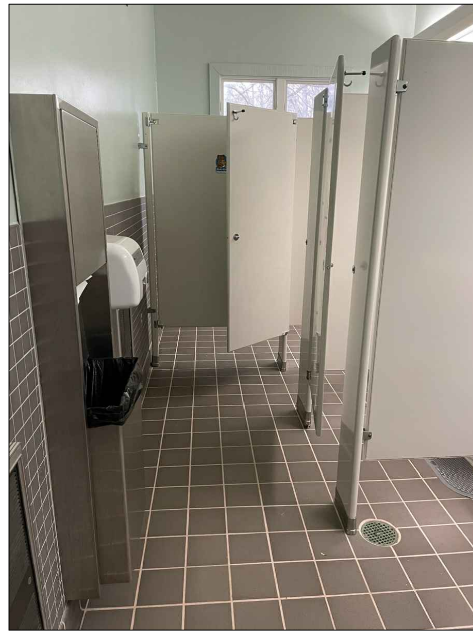
4 TYPICAL EXISTING CONDITIONS A1.1 NO SCALE
