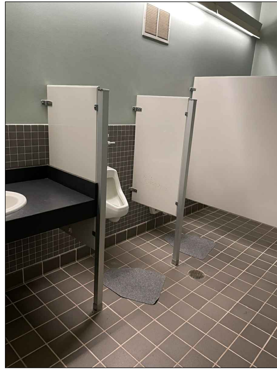
3 TYPICAL EXISTING CONDITIONS A1.1 NO SCALE
