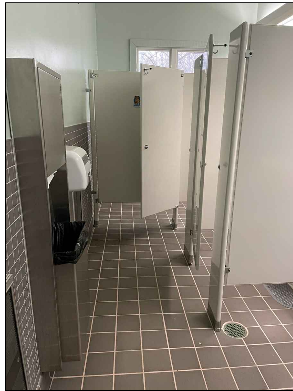
4 TYPICAL EXISTING CONDITIONS A1.1 NO SCALE
