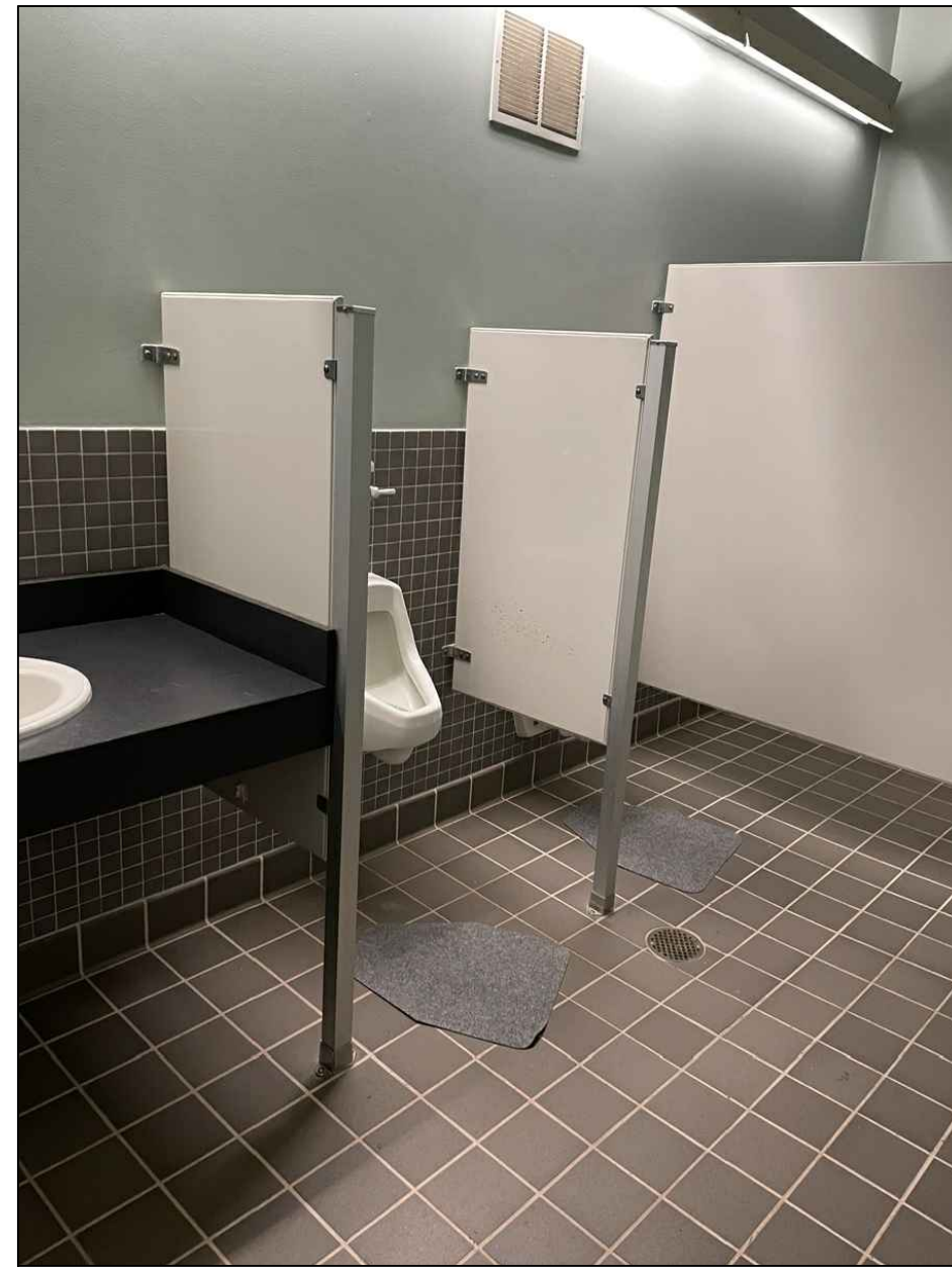
3 TYPICAL EXISTING CONDITIONS A1.1 NO SCALE
